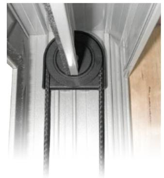
Pre-stretched, engineered rope runs through the counter balance pulleys. These rotate on sealed roller bearings, ensuring unparalleled ease of use, strength & durability
